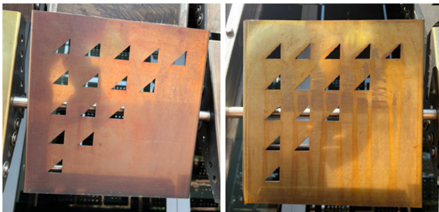
Figure series 28: Images of the Court's sun screens before and after they were cleaned, showing saturation of the patina, ranging from a golden-yellow to orange. Acidic rain has left watermarks on the sun screens but has not corroded the surfaces of the screens.
