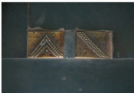
Figure 6: The Court's stair nosings designed by Jabu Nala are based on the patterns often found on ukhamba (traditional Zulu beer pots).
