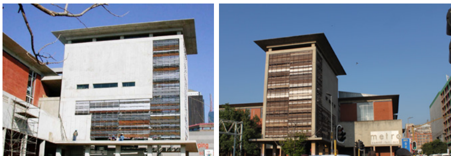
Figure series 30: The sun screens at the Metro Mall taxi rank in downtown Johannesburg when first installed (left), and in their darkened condition in 2022 (right).
