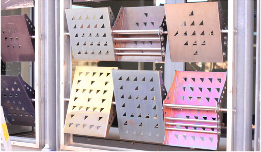
Figure 27: Each screen measures 29 x 28.5 cm. In some instances, the screens measuring 29 x 28.5 cm would leave excessive space at the base of the frame; an alternative dimension for 54 screens that measure 35.9 x 28.5 cm was used on the bottom layer of 22 frames.
