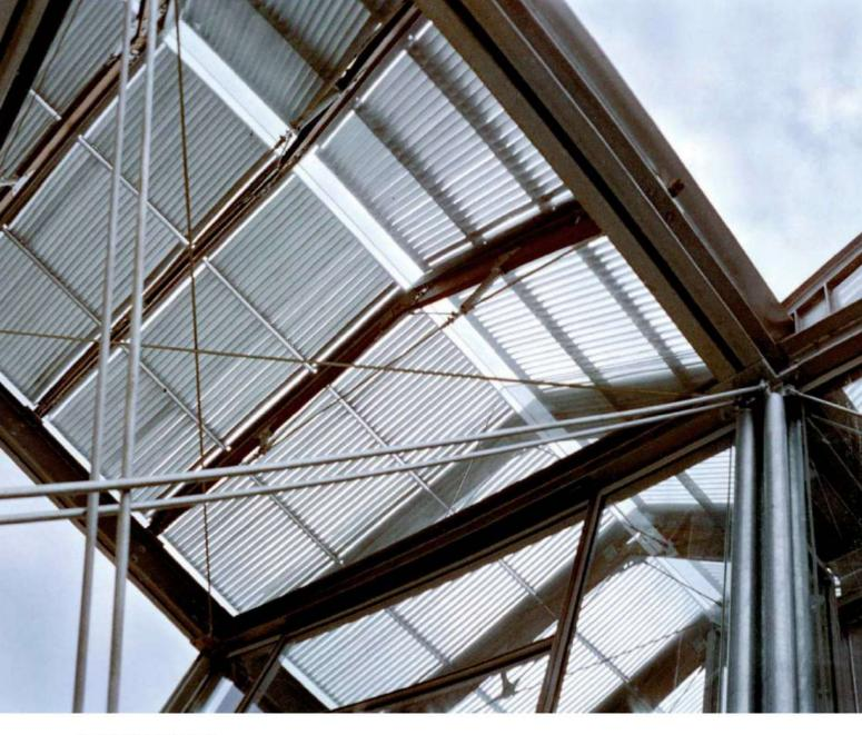
Lift housing showing cross bracing and internal steel columns. The glass structure is protected from direct light by steel shading.
