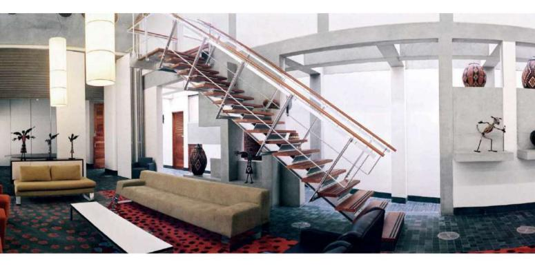
Above The staircase in the Judges' Lounge follows the design of the staircases linking the Judges' Walkways and those in the Welsh Library. The stairs are braced by a steel spine running down through the centres of the risers, a device that allows the stairs to appear light and free-floating.
