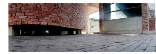
Left The southern wall of the Court Chamber showing the ribbon window and the recycled bricks from the Awaiting Trial Block
